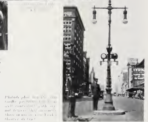
The man inside the tower has direct traffic control, he communicates the mechanism in the signal box. It is the hope of the experts to one day control all the traffic in New York from a single headquarters.
